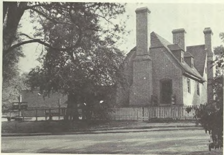
THE RECONSTRUCTED PUBLIC GAOL , Williamsburg, Va.; the original built by Henry Cary, Sr., 1703-1704. (Photo by Helen Estes Seltzer, 1977).
