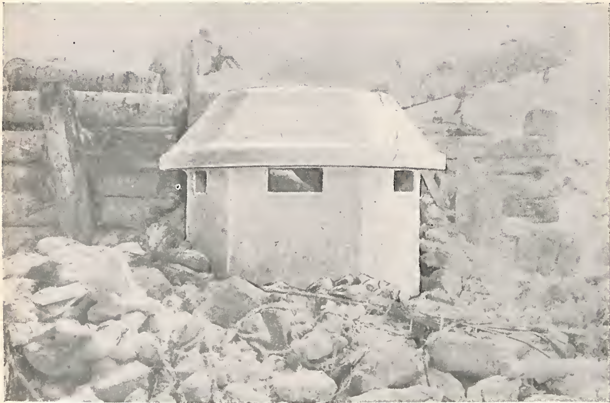
Figure 146. A concrete pillbox.
