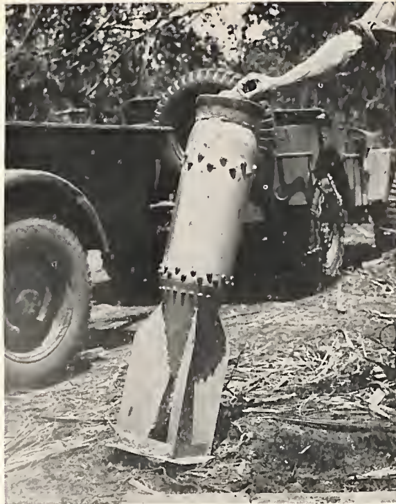
Figure 69. Model 99 (1939) 63 Kilogram General Purpose H. E. Bomb.
