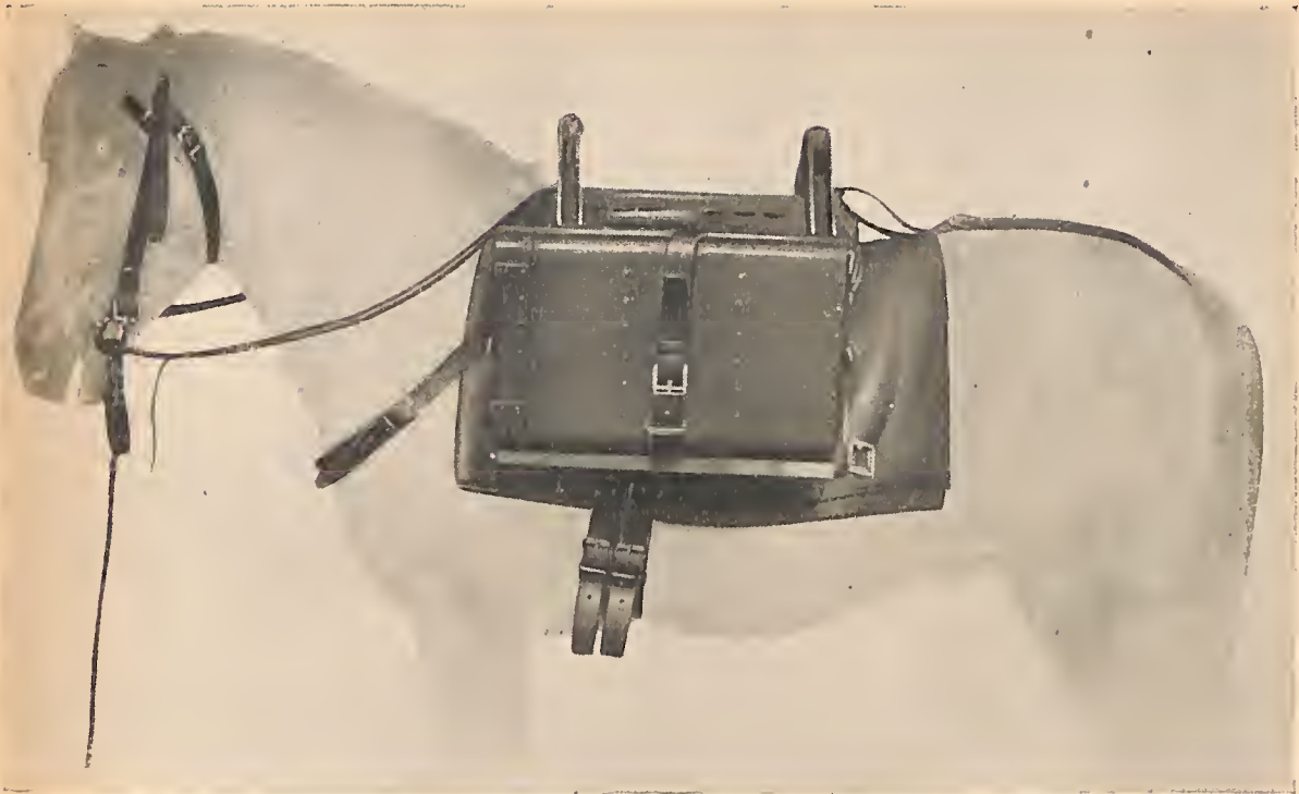
(Above) Figure 334. Method of fastening ammunition chest to pack saddle.
