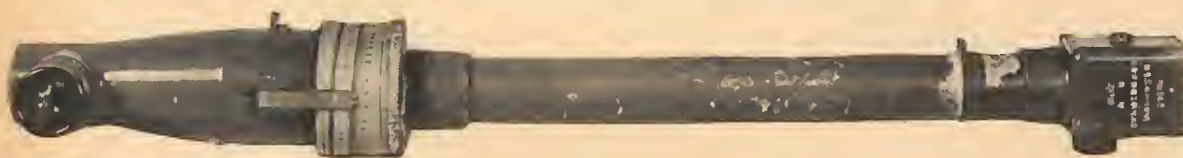
Figure 286. Model 92 (1932) 40-cm base range finder is calibrated for measuring ranges up to 1,500 meters (1,640 yards). It is a coincidence type of range finder with a 4\times magnification.
