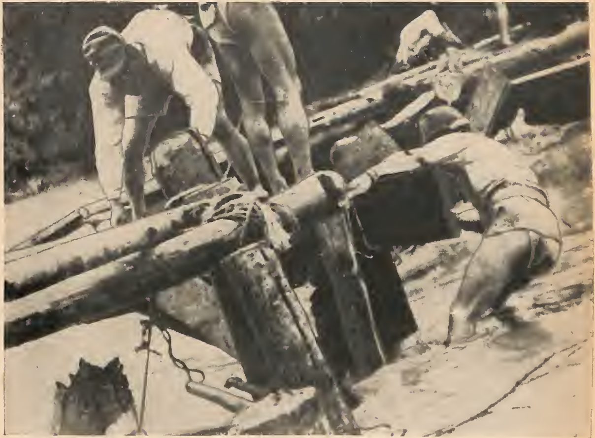
Figure 381. Improvised trestle bridge.
