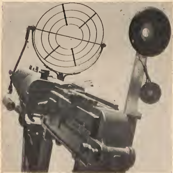
Figure 306. Front and rear antiaircraft sights mounted on the model 92 (1932) 7.7-mm machine gun.
