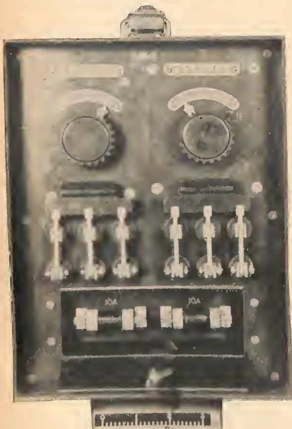
Figure 374. Battery charger, front view, showing controls.
