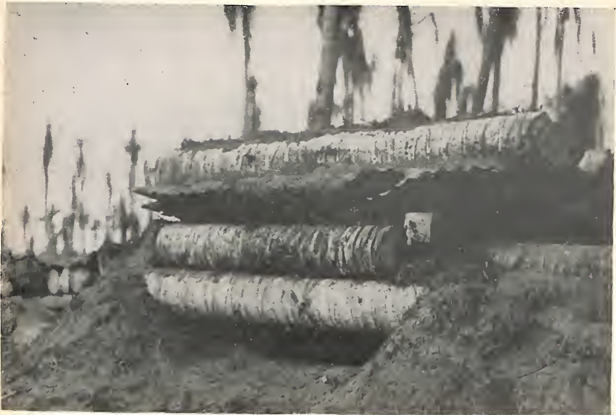
Figure 143. Exterior view of pillbox.
