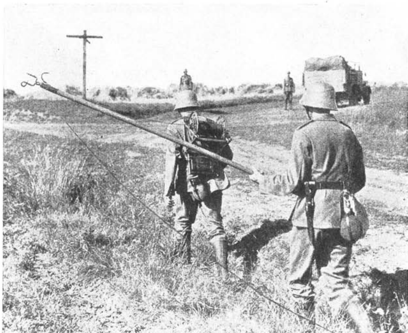
Figure 145.—Reeling out field wire.
