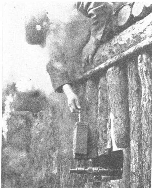
Figure 120.—Method of blowing a portal.
