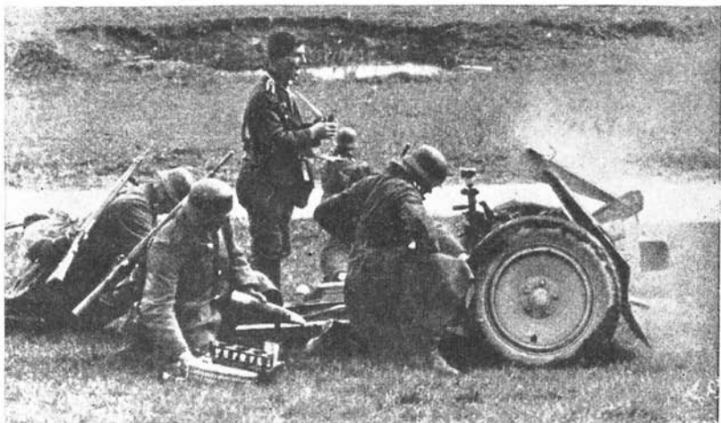
Figure 54.—75-mm infantry howitzer ( I.I.G. 18 ) mounted on carriage with rubber wheels.
