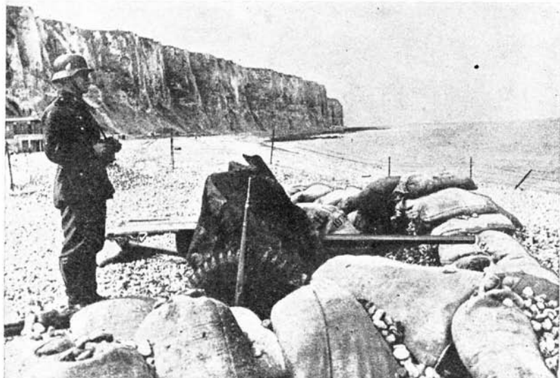
Figure 191.—Gun emplacement on a beach protected by barbed wire.
